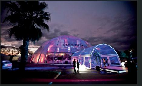
It has some impressive loading capacities with 3000kg per arch – which is more than 20 times greater than a standard marquee or temporary structures loading capacity, making the Igloo the perfect structure for an event with a large production element such as a concert or festival.
